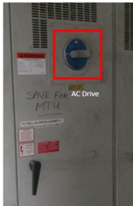
Figure 52: AC drive power switch [3]
