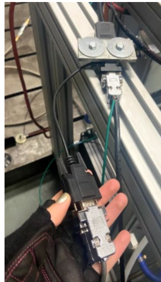
Figure 78: Connecting DB9 cable to inverter cart
