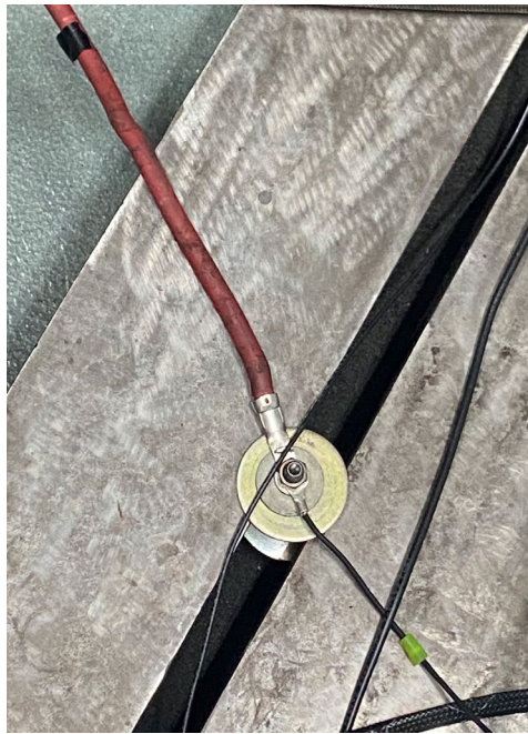
Figure 31: 9/16" grounding bolt for inverter to bedplate
